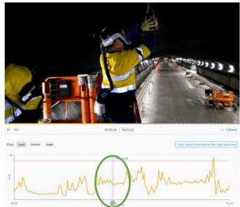
The above charts demonstrate the difference between the load on the arm when overhead drilling with two different types of drills. The first drill (red circle) increased the load on the arm by 34% compared to the second drill (circled in green).
